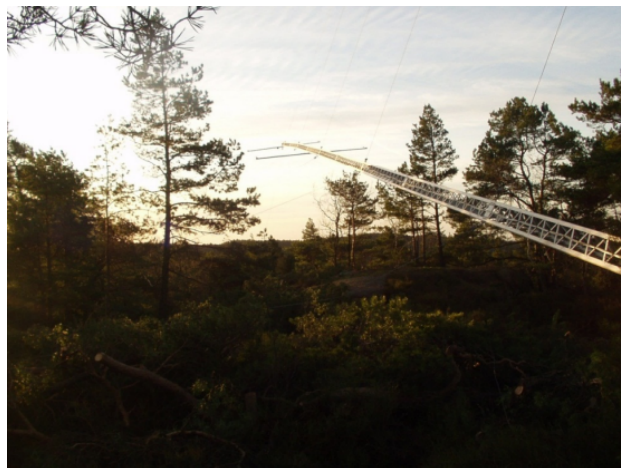
Figure 6.3: Installation of the meteorological mast.
