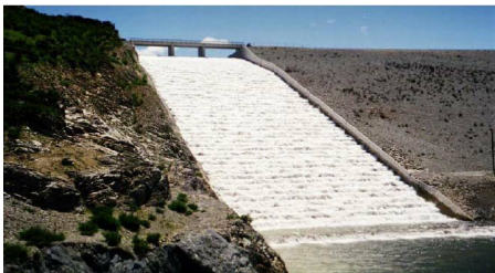
(a) Stepped Spillway 5
