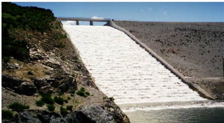
(a) Stepped Spillway 3
