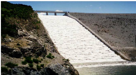
(a) Stepped Spillway 1
