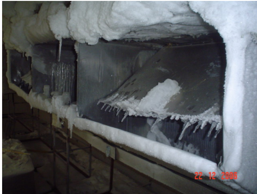
Figure 6. Duct opening in the middle refrigeration unit showing an aluminum plate inside the duct
