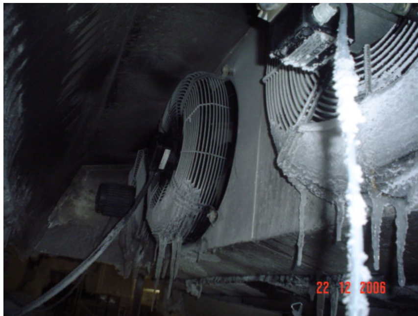
Figure 7. Back side of a refrigeration unit showing the three blowers which blow the air across the evaporator
